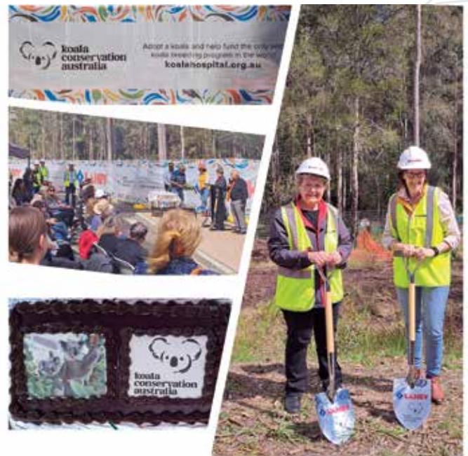
The Sod turning ceremony to mark the start of the build of the breeding facility.
